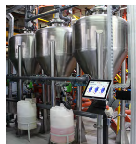
Top: RecondOil recycles lubricating oil at SKF's ball-bearing plant in São Paulo state, Brazil. Above: the RecondOil process, which was first used in Sandvik, Sweden, can be employed in many industrial plants that use lubricating oils
